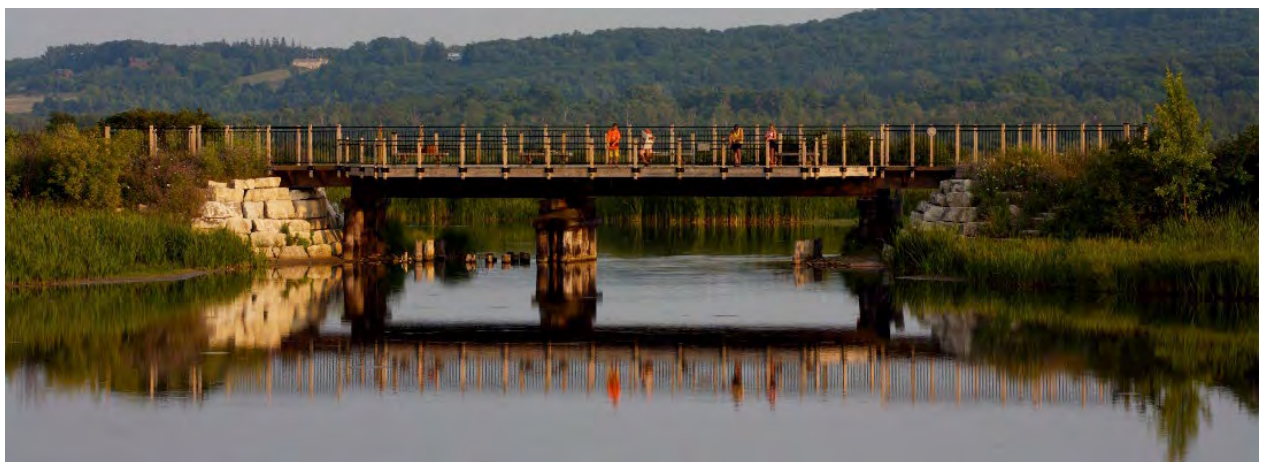
Betsie Valley Trail Bridge
