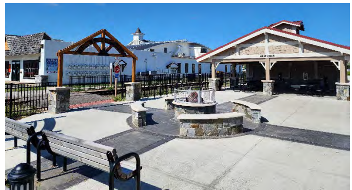
Gaylord Gateway Trailhead for the NCST
