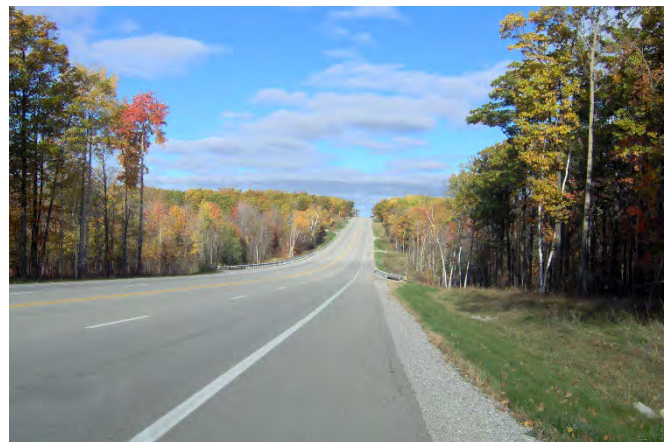
Paved Shoulder Along US 23 near Black River
