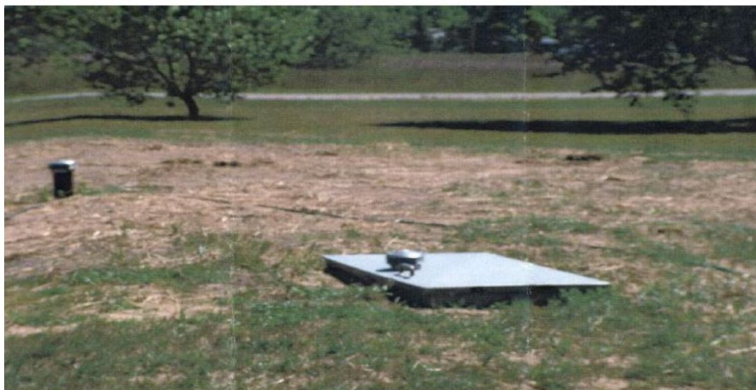
Figure 17. GTB Tribe Storm Shelter Entrance
