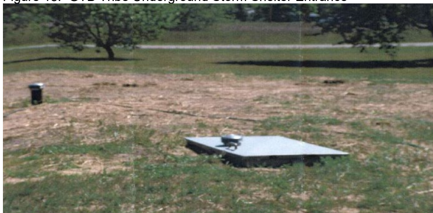
Figure 18. GTB Tribe Underground Storm Shelter Entrance
