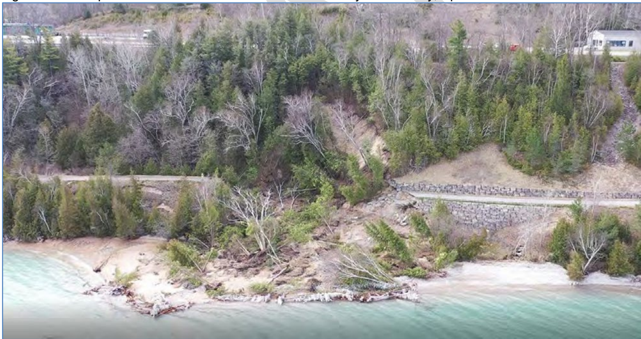
Figure 38. Collapsed Portion of the Little Traverse Wheelway in Petoskey, April 13 2020
