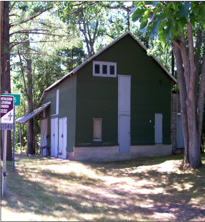
Historic Blacksmith Shop near County Road 675, north of Glen Arbor
