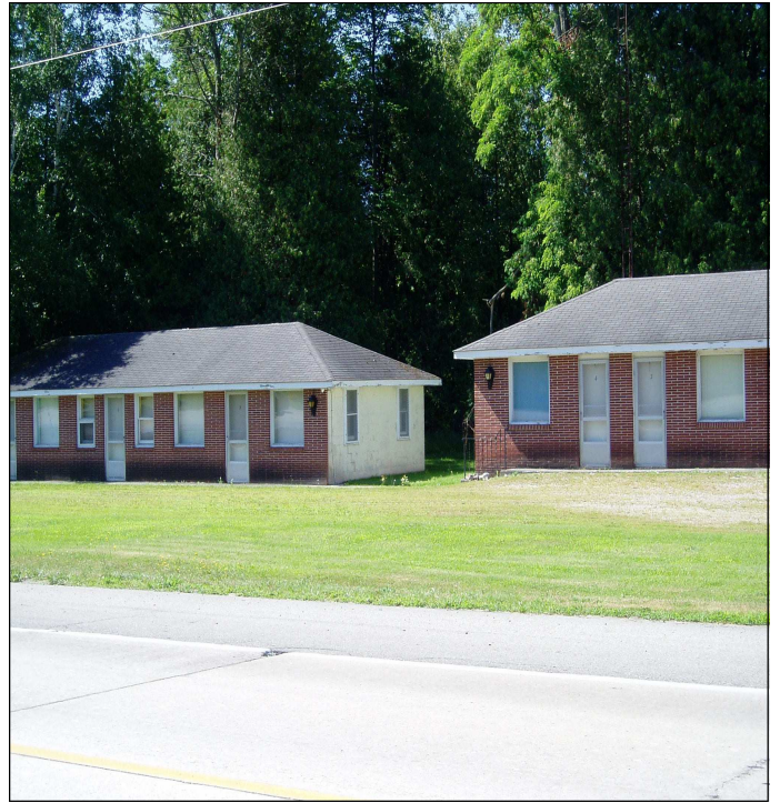
Old highway motel—not in operation
