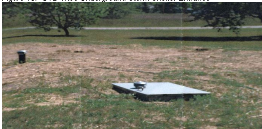
Figure 18. GTB Tribe Underground Storm Shelter Entrance
