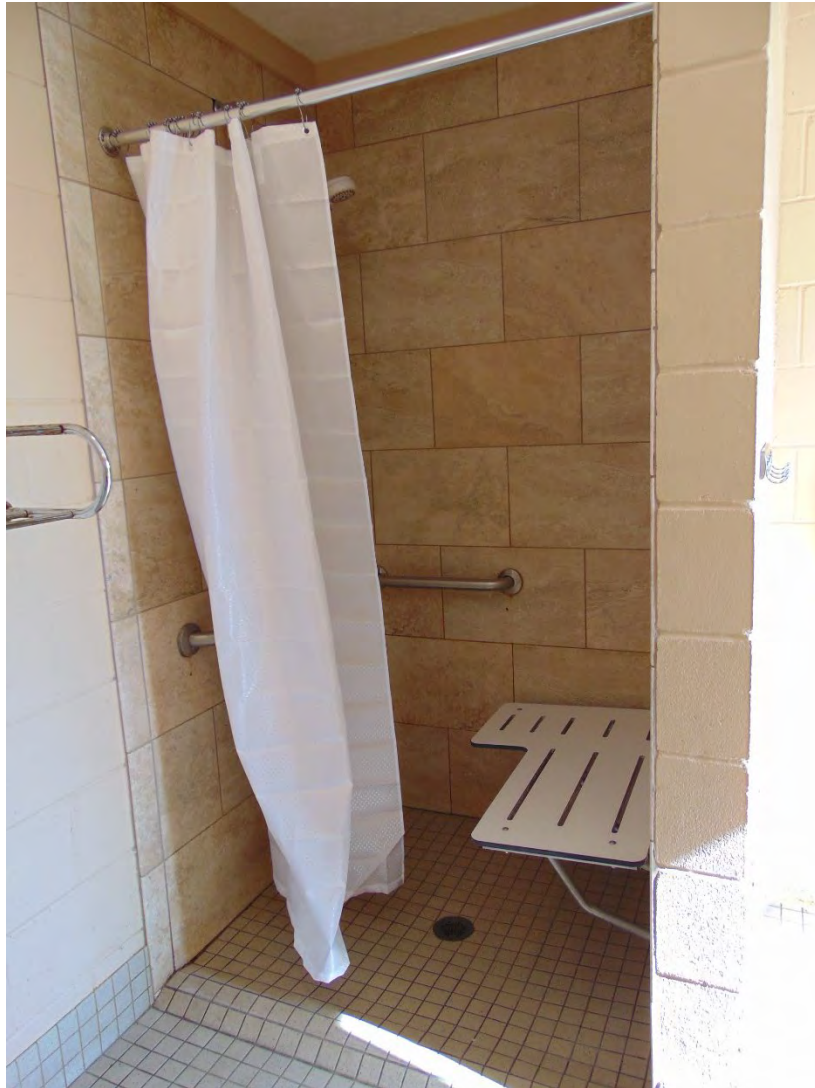
Interiors of renovated and ADA Accessible bathrooms.
