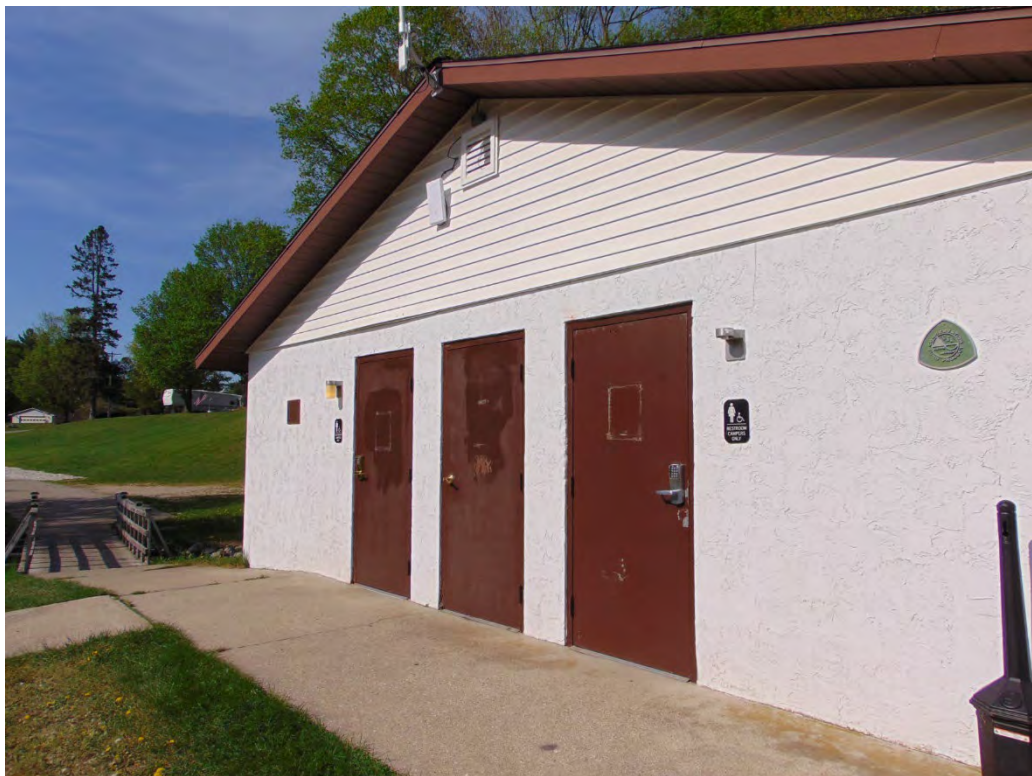
Thurston Park bathroom building.
