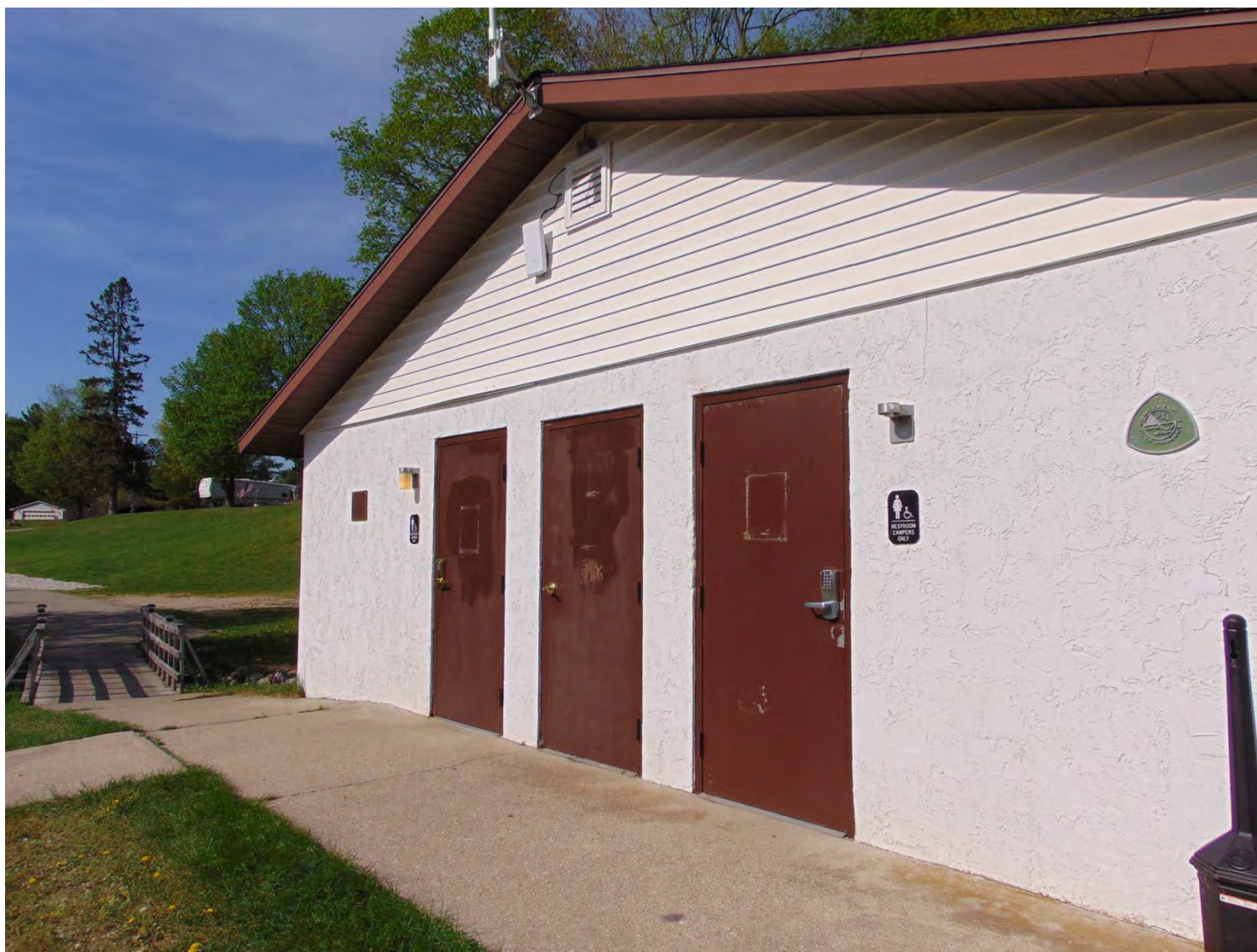
Thurston Park bathroom building. Notice the ADA accessible signage and door handles, and the LWCF Recognition plaque.
