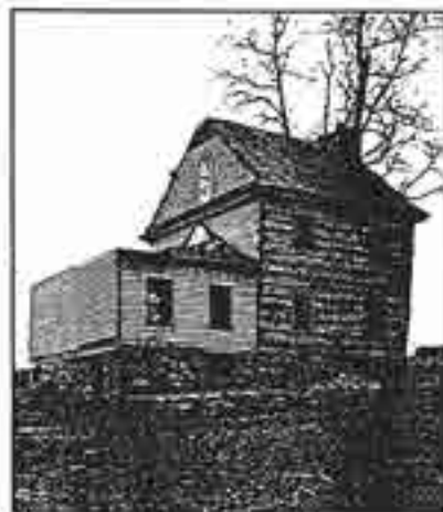
The second photo should be a perspective of the rear and other side of the building. These two perspective shots now comprehensively document the exterior of the structure. The slope of the hill dictated a vertical view to maintain perspective control. The James Stewart House.
