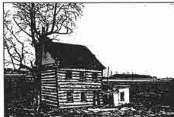
If you were allowed only one photograph to document an historic structure, the best choice would be a perspective showing the front and one side of the building. The James Stewart House, circa 1748, Lancaster County, Pennsylvania. All photographs taken by David Ames unless otherwise noted.
